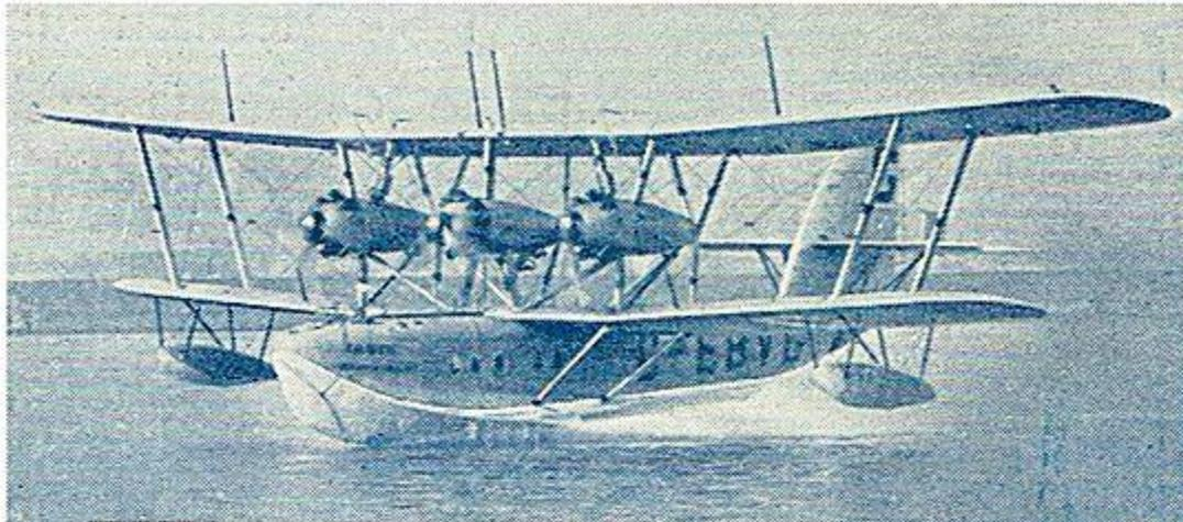
*For the Genoa-Alexandria section of the Air Route to India, SHORT "CALCUTTA" flying boats are employed. These boats are of all-metal construction, and are fitted with BRISTOL "JUPITER" engines. As in the boat itself the construction is in one aluminium alloy (DURALUMIN), so in the engines the castings are mainly of another aluminium alloy (ALPAX).*
