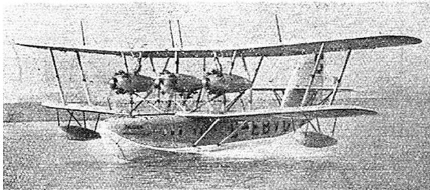
The SHORT "CALCUTTA" all-metal commercial flying boat, constructed substantially of aluminium alloys (Duralumin and Alpac).
